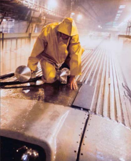
ABOVE: In 1966, the new Metroliner cars were already under construction at Budd's plant in Red Lion while the high-speed test program was underway. This completed carbody is being tested for water-tightness. JIM DIFFENDERFER, BOB WATSON COLLECTION
